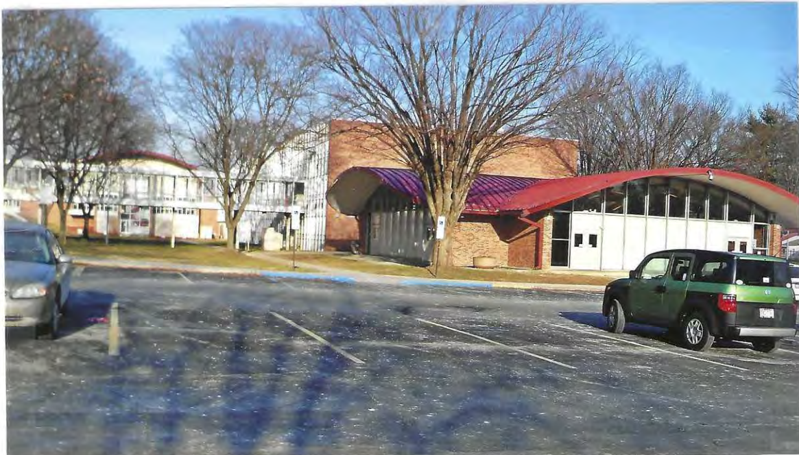
EASTERN WING, BRIDGE, AND CAFETERIA
