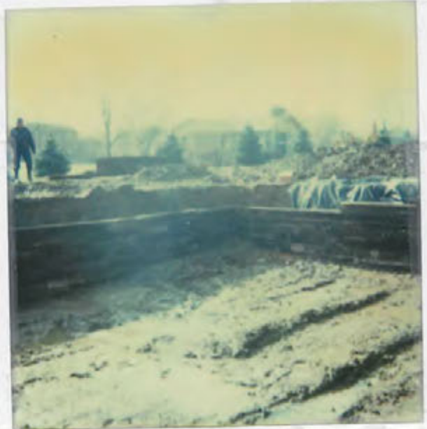
LAKE HOUSE BLOCK WORK, 1976
