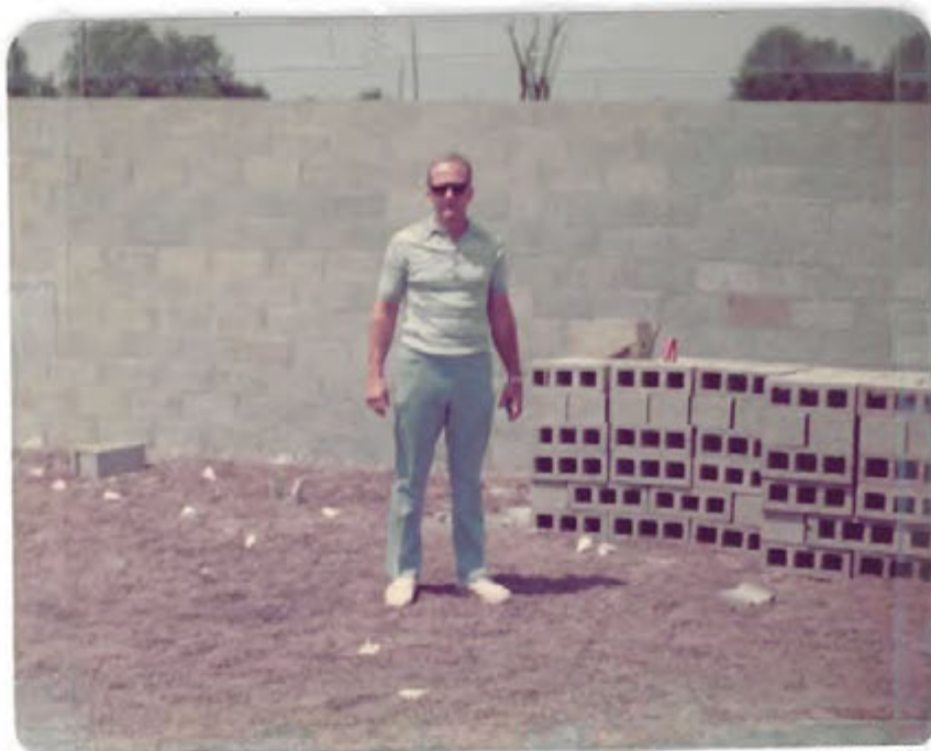
ED SR AND BLOCK WORK (August, 7, 1976)
