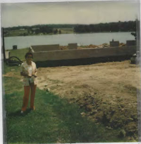
1976 Lake Latonka Block work
