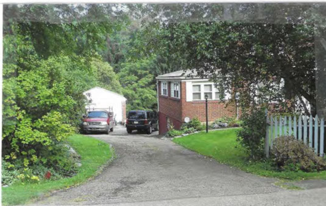
house and garage at 1656 Charlton heights Road before the explosion on October 12, 2013
